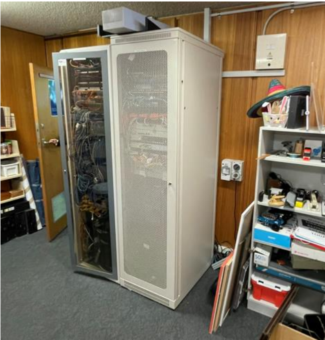
Figure: Existing campus distributor racks
