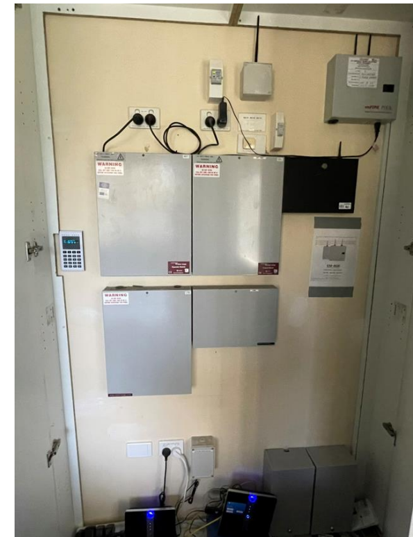
Figure: Existing security headend
